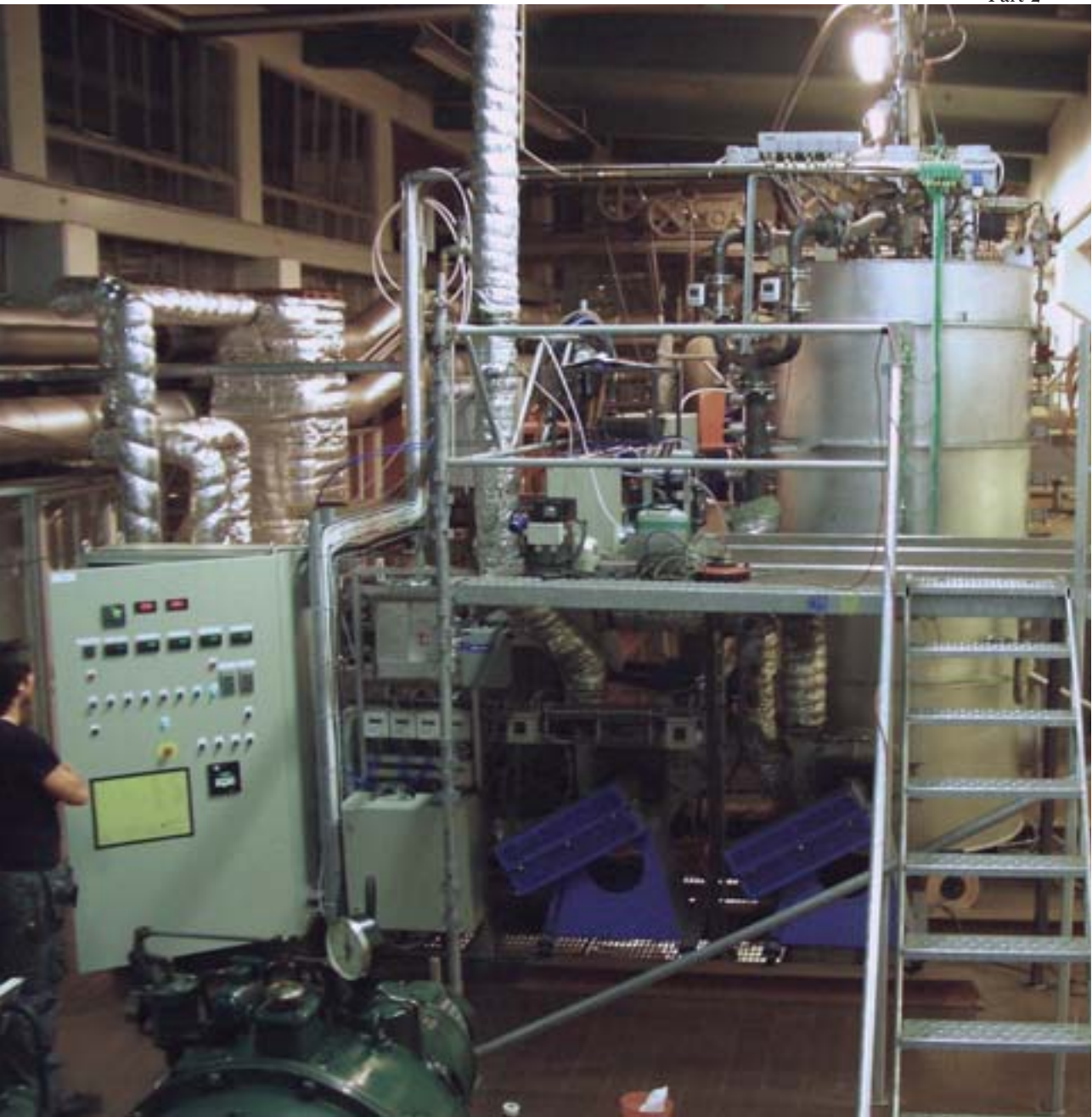
Front side of the Chalmers 100 kW oxy-fuel combustion test unit showing the top fired 3.0 meters high combustor. In the background to the left the fabric filter can be seen with the surrounding piping system.
