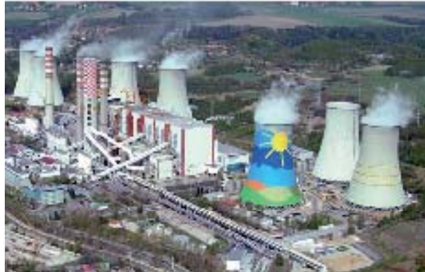
Cooling towers with their pillars of steam
